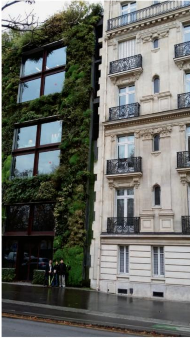
Figure 3.6. The vertically planted green wall on the facade of the Musée du quai Branly, designed by Patrick Blanc, inserts green plants into this highly urbanized setting. The adjacent building, although it lacks living organisms, subtly enhances this biophilic quality by virtue of its organic shapes and forms, natural materials, and natural geometries. The juxtaposition of all these elements elicits the human affinity for nature.
