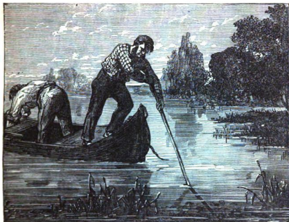
POLE SEEMING TO BE BENT.
