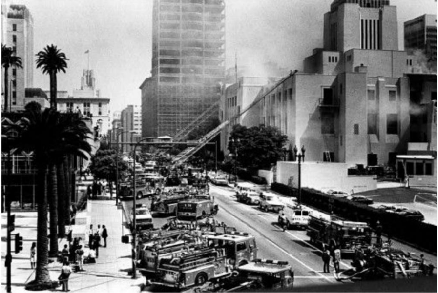
The fire as seen from Fifth Street
