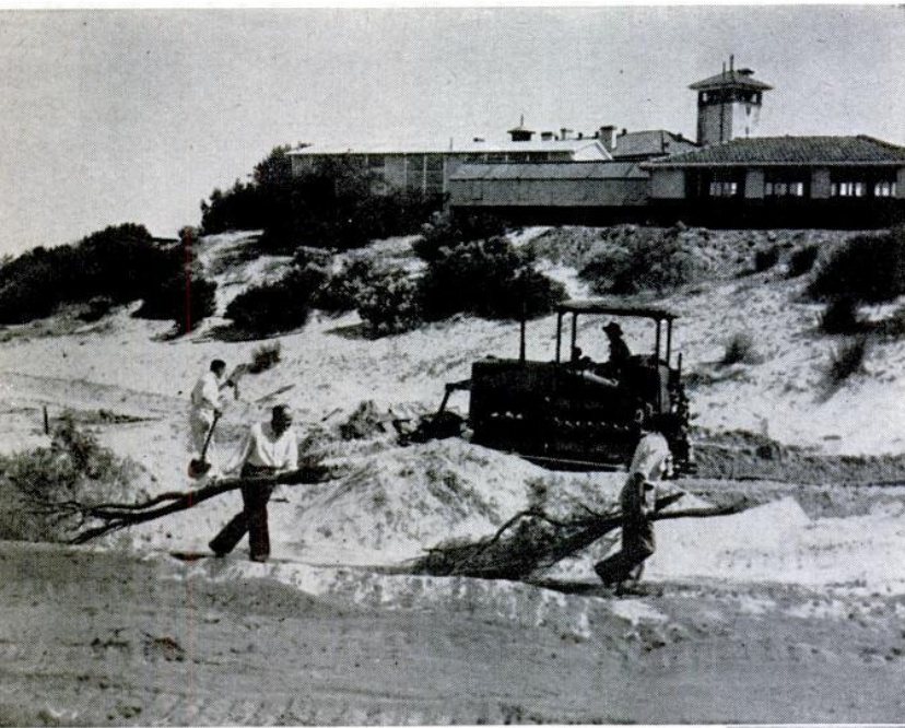
Men at work: members of the Rotary Club give their labor to help build tennis courts for Bunbury High School. They had discovered this need by a community survey.
