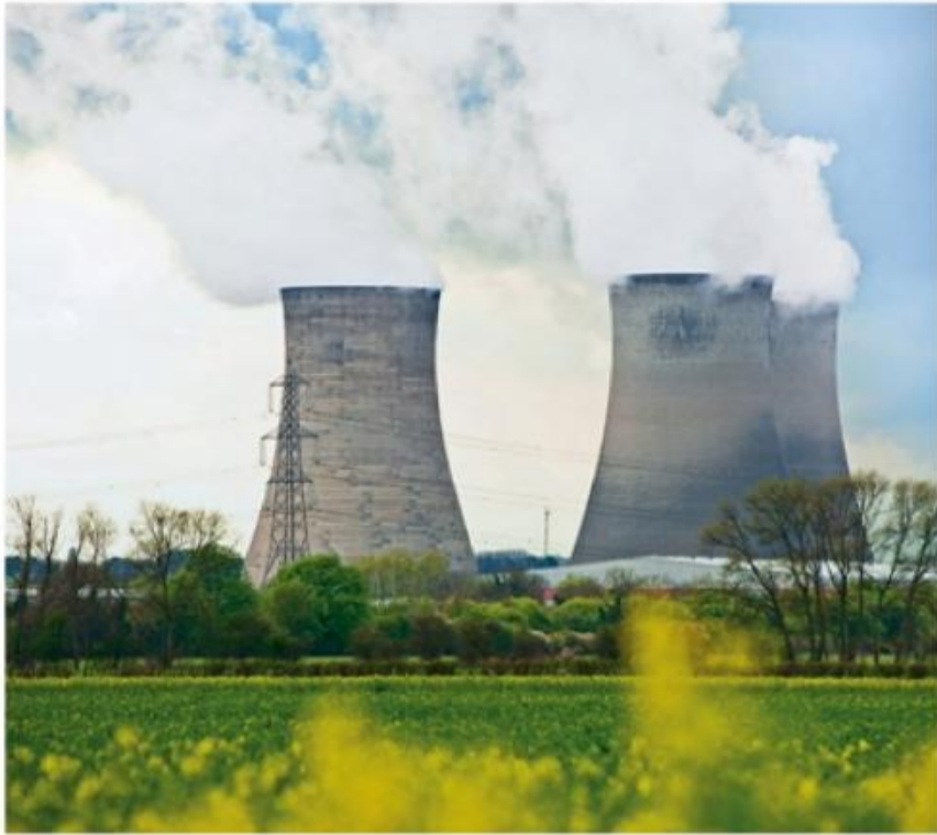
Like many power stations, this one in Didcot, England, uses cooling towers whose curved outline is a parabola.
